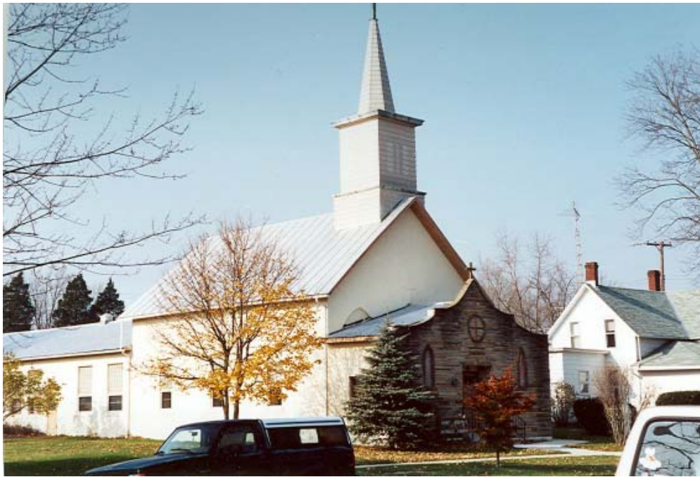
St. Joseph Church, LaRue, after the additions in front and rear.
