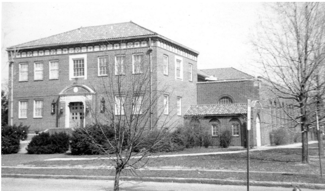
Rosary High School, looking east from Berkeley Road.
