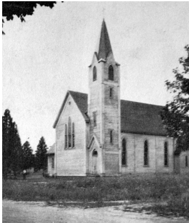
The original St. Sylvester Church, built in the 1860s. The tower was added in Father Slevin's time. It burned down in 1929.
